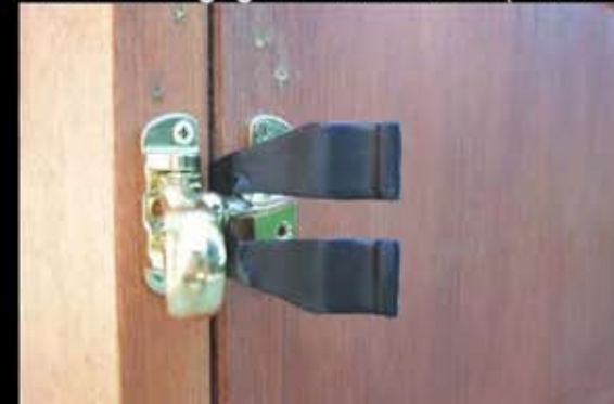
Latch Disengaged- Interior View (Photo 3)
