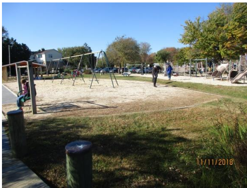
1. Install area for climbing structure
