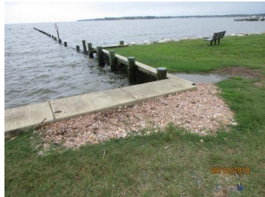
7. Repair the seawall/bulkhead sinkhole
