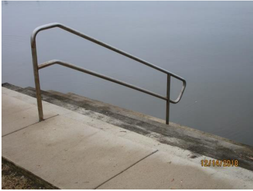
3. Reinstall swim area step rail
