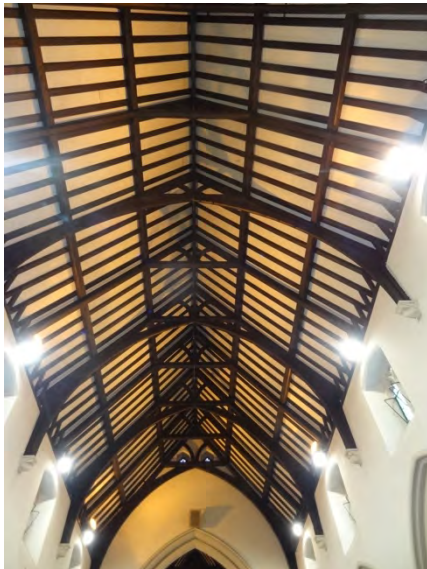
Nave ceiling and roof structure
