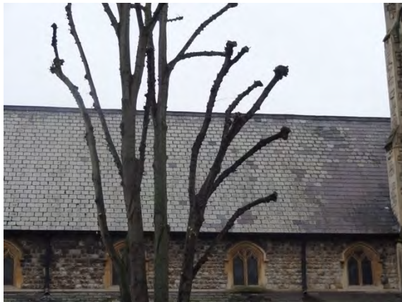
Nave roof north pitch
