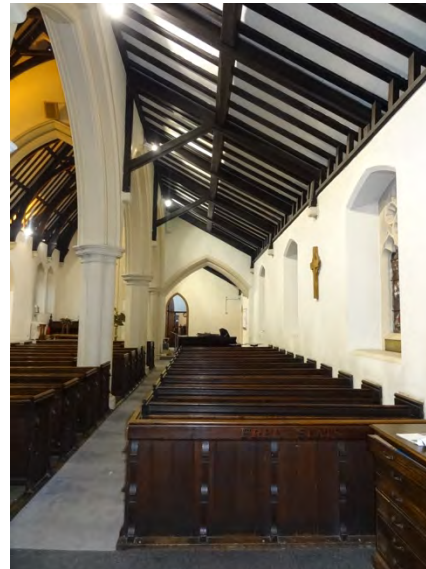
Aisle and aisle roof structure
