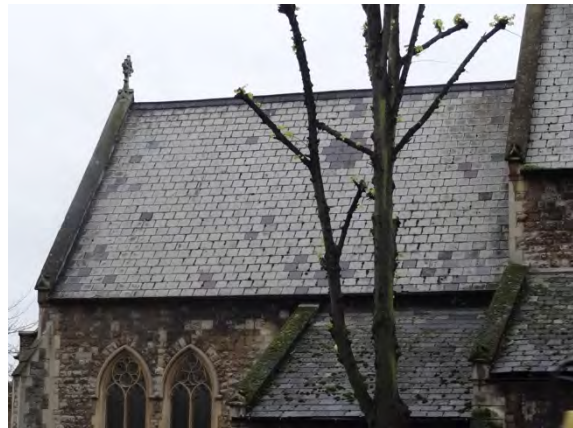
Chancel roof north pitch
