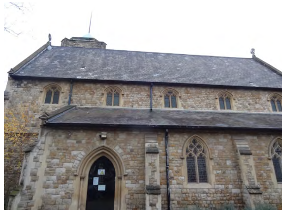
Chancel and aisle roofs south pitch
