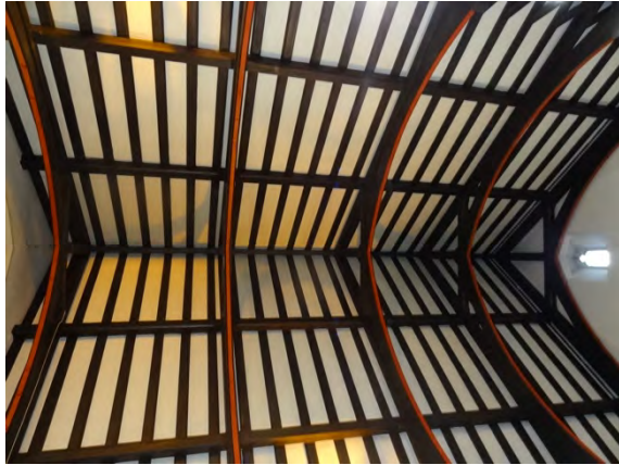
Chancel ceiling and roof structure
