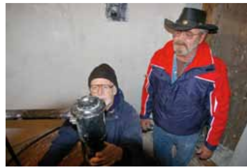
Russ Santoro, left, and Steve Scyoc, ICC, on lighthouse renovation project
