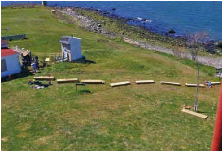
Scouts place new walkway between the stairs and the bunk house
