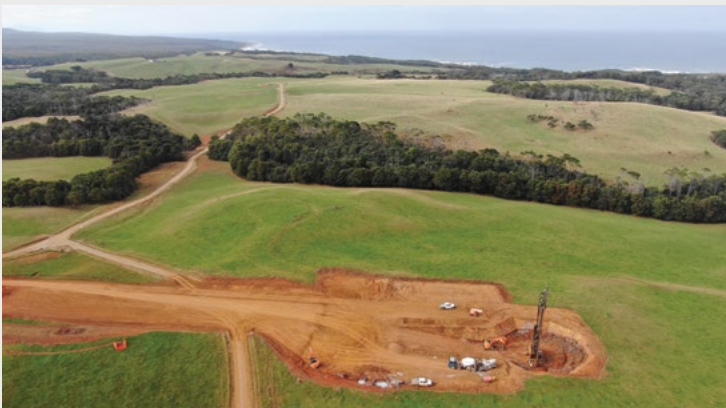
Aerial view of construction works for a wind turbine foundation
