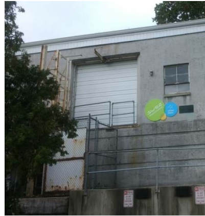
Central Avenue Pump Station (CAPS), Yonkers, NY
