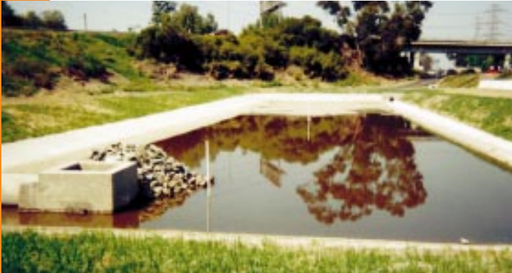
One of the detention basins designed and operated by Brown and Caldwell to treat storm water for Caltrans. The company designed ten full-scale storm water treatment units for the agency and has been operating eight of them, six of which Brown and Caldwell also built. They include an oil/water separator and units with various types of filters.
