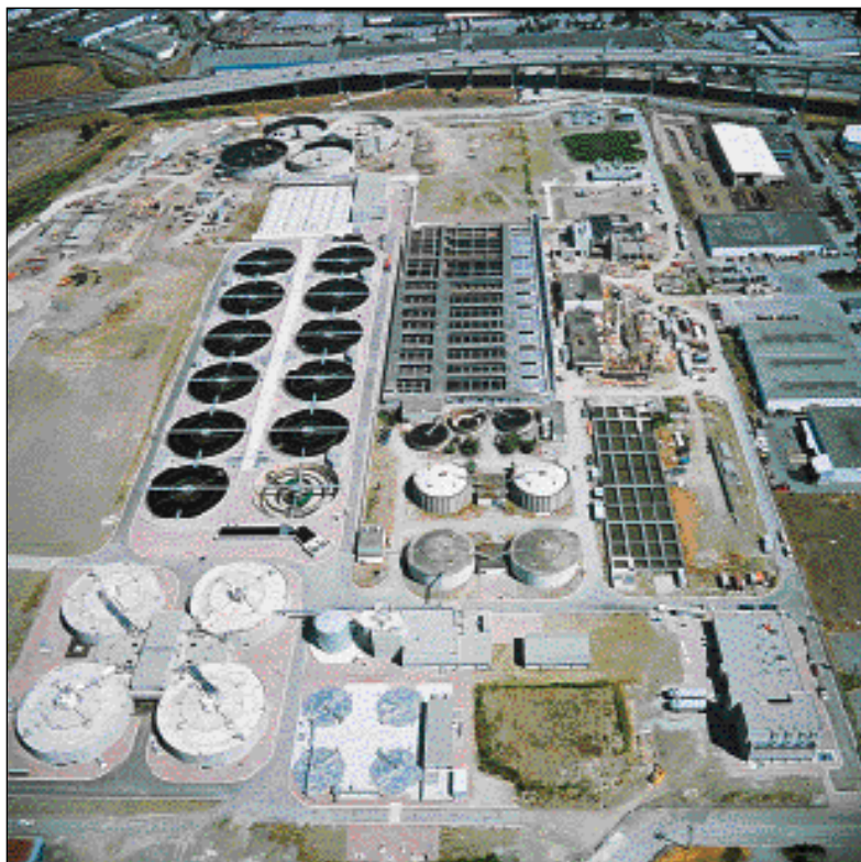
The Annacis Island wastewater treatment facility, scheduled for start-up this summer, will be the largest and most technically advanced trickling filter/solids contact plant in the world. Shown (clockwise from lower left) are four new thermophilic digesters; 12 secondary clarifiers; four solids contact tanks and four trickling filters; 13 primary sedimentation tanks, three gravity thickeners, four digesters, and chlorine contact tanks from the original plant; new influent pumping station and operations and maintenance buildings under construction (upper right); the new cogeneration building (lower right); the heat recovery building; and four dissolved air flotation thickeners.
