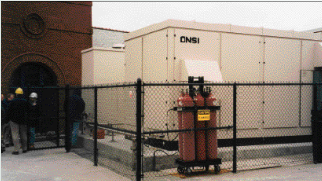
The fuel cell that was part of a demonstration project at the Deer Island wastewater treatment plant in Boston. Eugene Appel, principal engineer for the Portland, Ore., Bureau of Environmental Services, is among the group at left examining the fuel cell.
