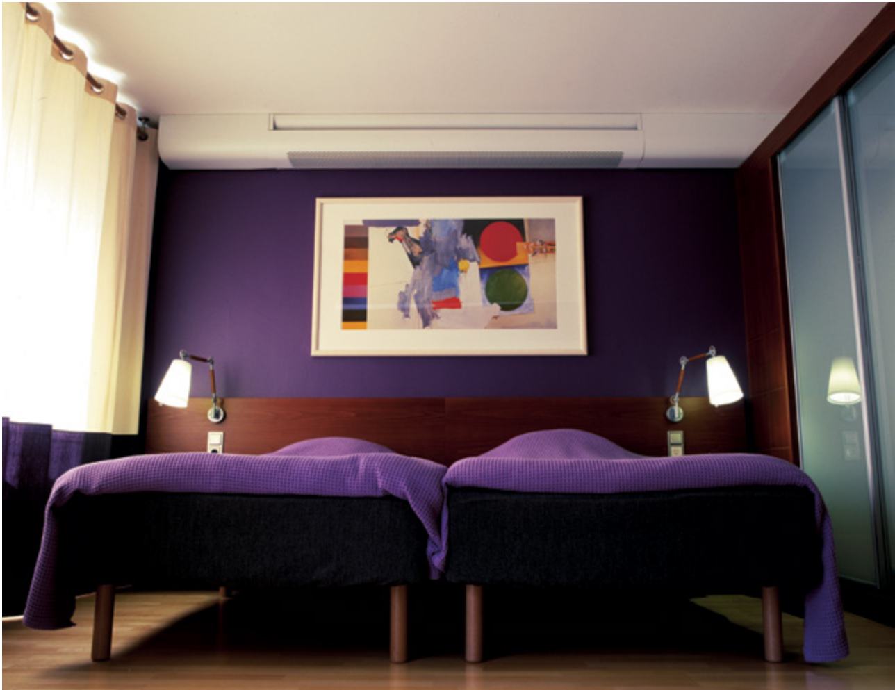
Picture 1. Plafond is suitable when the ceiling should be free from equipment.
