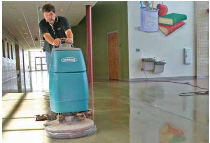
Auto-scrubbing with Consolideck LSKlean or Consolideck DailyKlean is the recommended way to perform maintenance cleaning of Consolideck finished concrete flooring.
