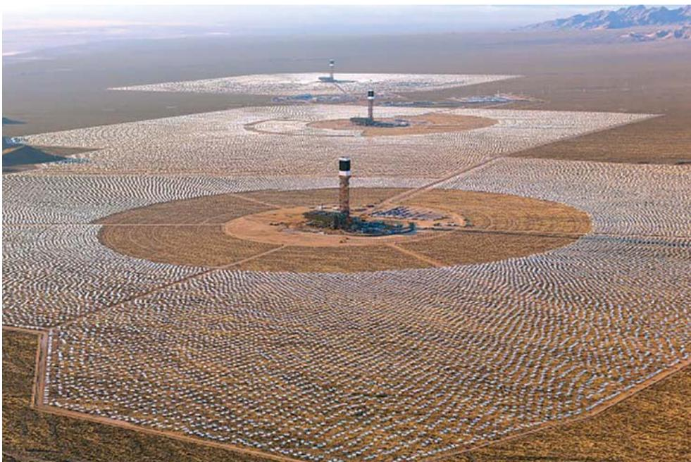
At the Ivanpah Solar Electric Generating System, more than 300,000 computer-controlled mirrors beam concentrated sunlight to three 460-ft-tall towers. (Photo courtesy NRG Renew)
