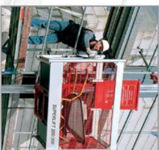
Platform – The swivelling platform enables use on narrow sites.
