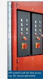
VIF control unit for fast access, e.g. for rescue personnel
