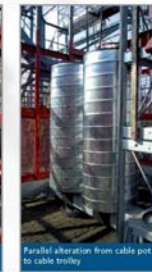
Parallel alteration from cable post to cable trolley
