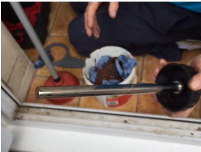
Central magnet before cleaning
