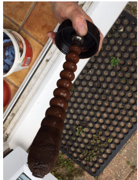
After cleaning just one radiator
