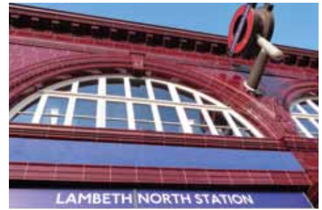
Lambeth North Station Restoration Client: Transport for London
