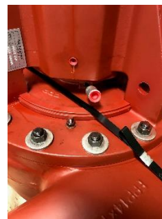
Remove Switch Cap
