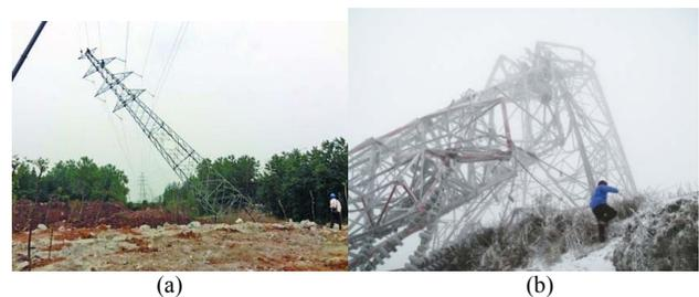
Figure 1: Tilted and collapsed tower
