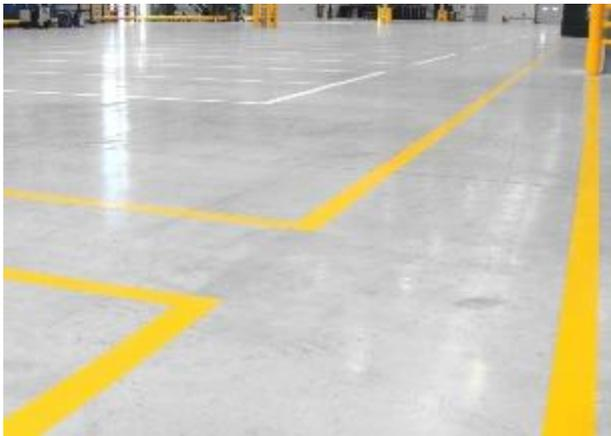
Even though this method of floor marking is called 'unprepared' we do require the concrete surface to be free from dirt, dust and debris before applying the paint. We may need to use a scrubber dryer, solvent and/or other material to help make it as tough as we can for you, but this is an additional item to be charged for.
