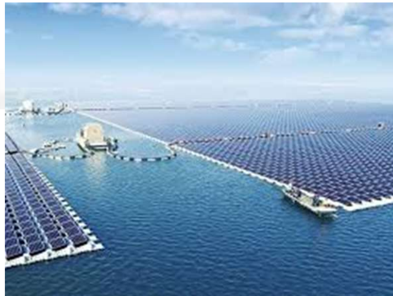
Floating Solar farm
