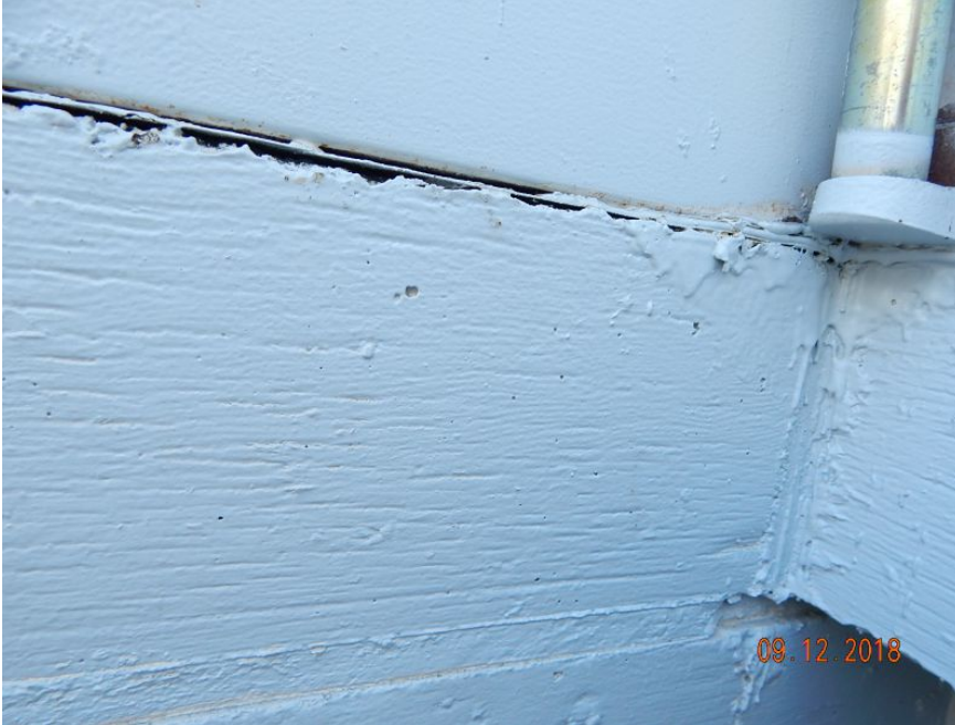
Reinforced Concrete Roof Deck
