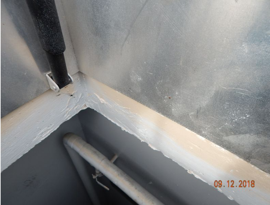
Reinforced Concrete Roof Deck
