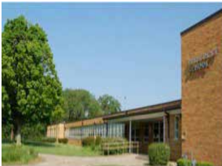
Hillcrest Elementary School
