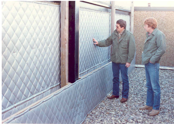
Outdoor installation shows the use of QAB-200-SM panels to line rooftop enclosure walls around noisy HVAC equipment.
