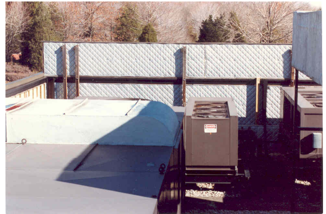
Outdoor installation shows the use of QAB-200-SM panels to line rooftop enclosure walls around noisy HVAC equipment.
