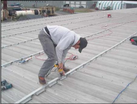
When retrofitting an existing metal building with a new "Metal-over-Metal" roof overlay, it is extremely important to address building code requirements that have changed since the building was originally constructed. Several factors should be considered during the planning process to ensure the existing building's roof and its new roof will perform for many years and will not be subject to catastrophic failures. These factors include:
