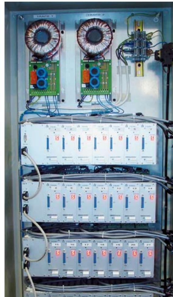
Modular control cabinet for 28 UHF elements, complete with low-voltage power supply.
