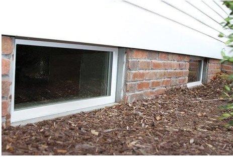
This window is at-grade.
