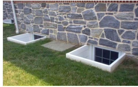
This window well is below grade.
