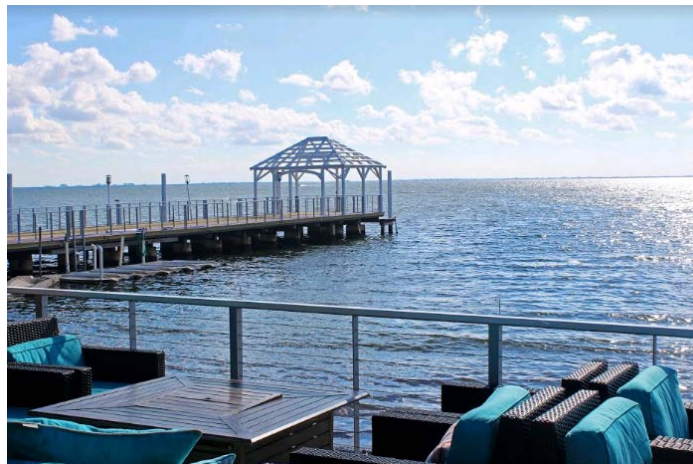
The newly-renovated 3,200-square-foot pier at The Godfrey Hotel & Cabanas Tampa
